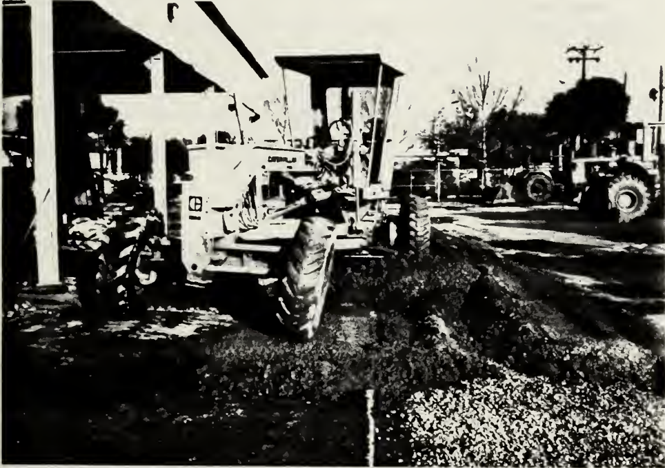
Figure 2.19 Grader Windrowing Wet Mixed Material
